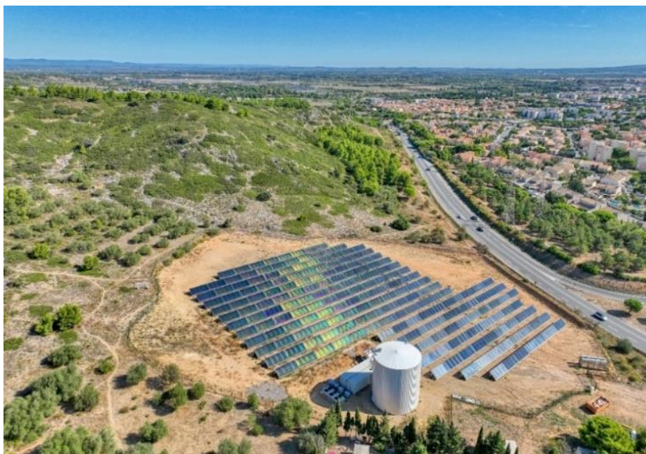
The NARBOSOL solar thermal plant, which supplies the district heating network of the French town of Narbonne.
