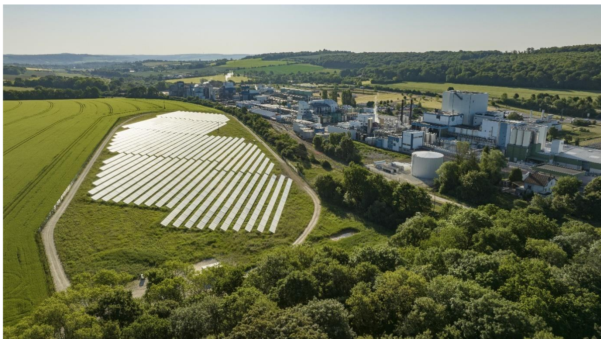
LACTOSOL Solar thermal plant, which supplies the Lactalis Verdun site ( Photos HD )
